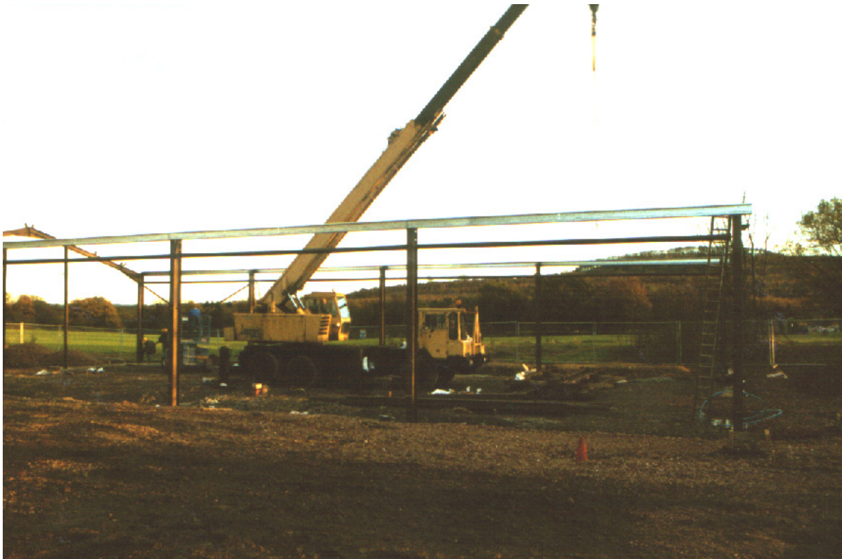
Construction of the Greenkeepers Accommodation, 2000
