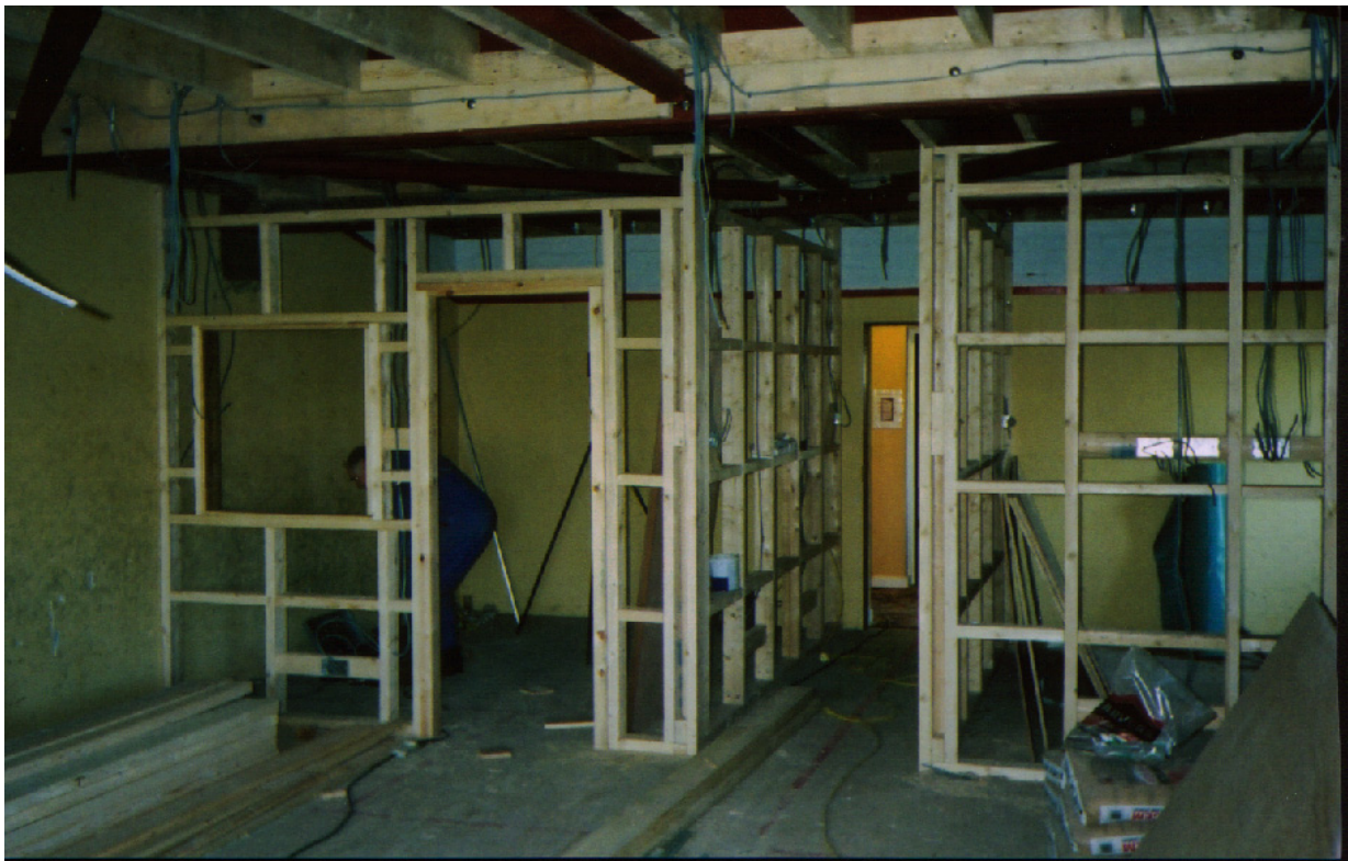
Conversion of No 4 squash court into the Pro Shop.
