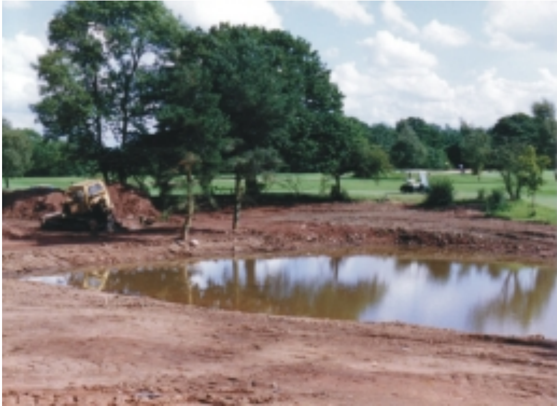
Construction of the Lake on 10 th – 2000
